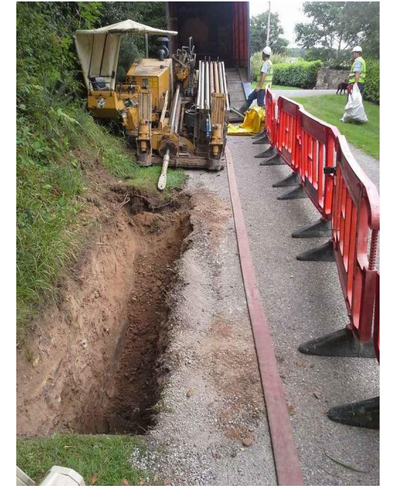
Image 2 : Typical Drilling Rig and Launch Pit
